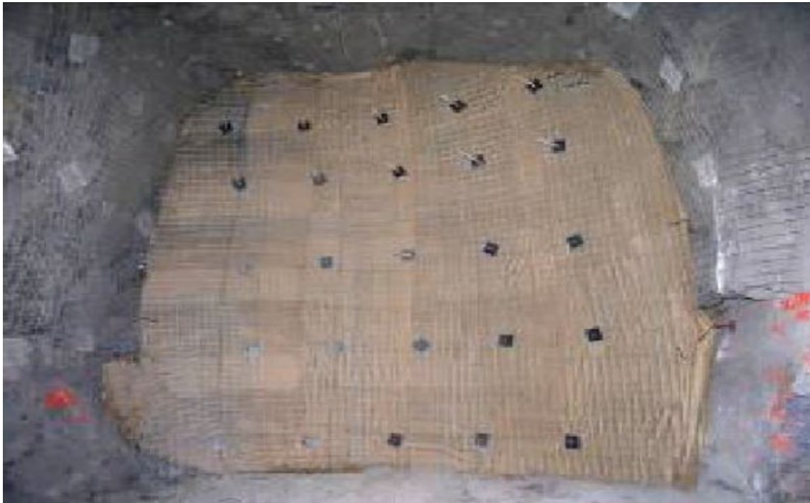
Figure 16.31 Paste Wall prior to Shotcrete Application (Minefill, 2022)
