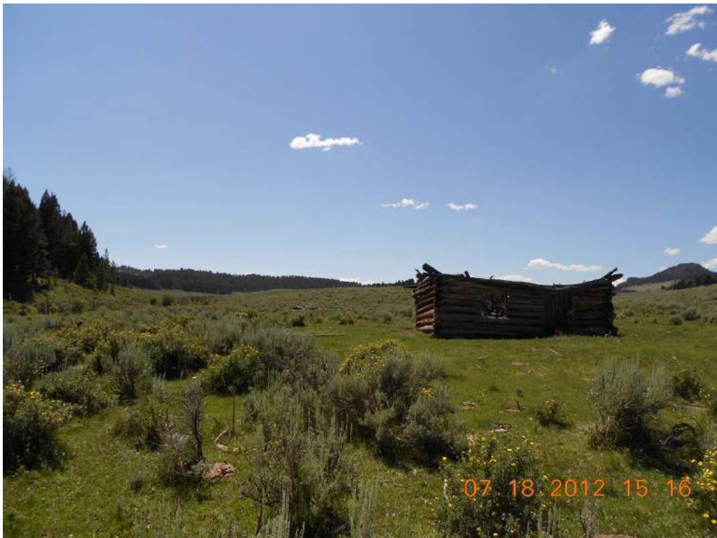
Site overview looking west
