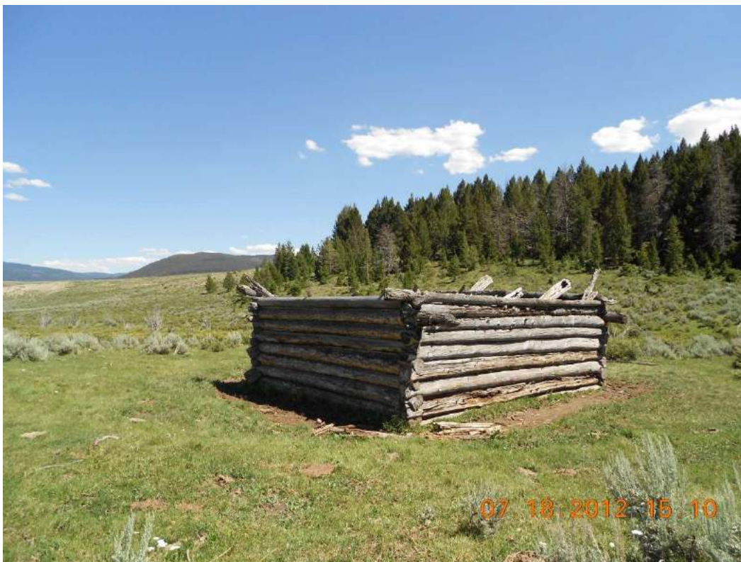
Feature 1. North and West elevations
