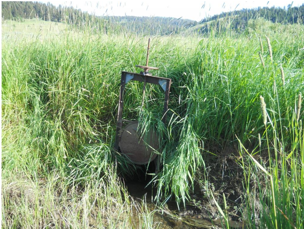
Ditch Gate, View to Northwest
