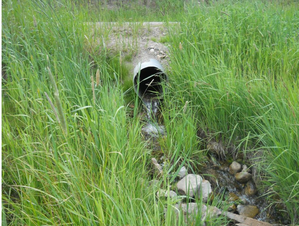
Road Culvert where Coon Creek Irrigation Ditch Begins, View to Southwest
